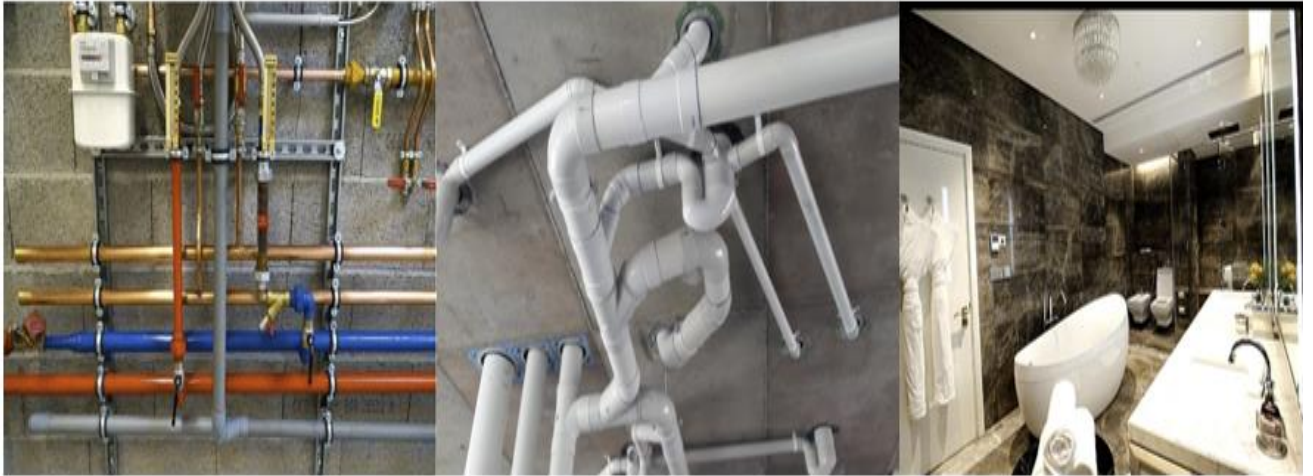
PHOTO : Plumbing and sanitary works
